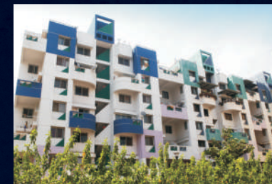
NAADBRAHMA 1 & 2 BHK Apartments @ Warje No. of flats 486
